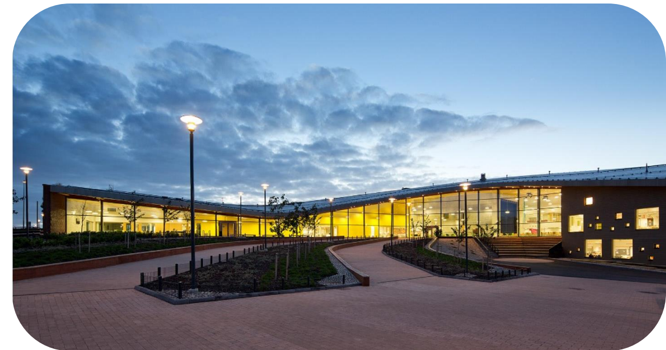
Figure 73. Large windows provide a panoramic view of the surrounding nature- Saunalahti School © Reino Tapaninen
